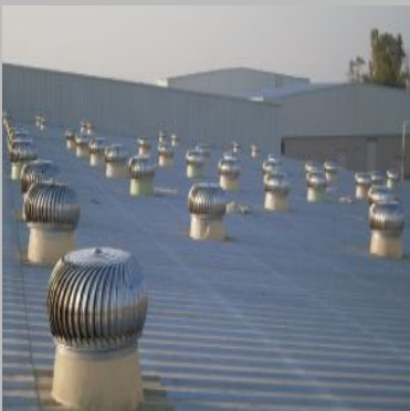
Turbine Air Ventilator
