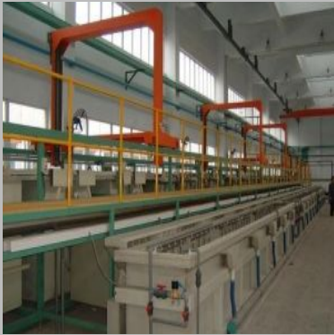
Zinc Electroplating Plant
