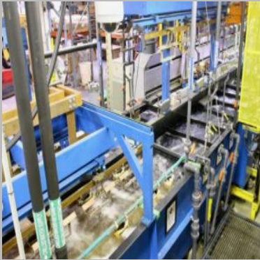
Tin Plating Plant
