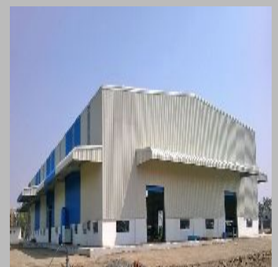
Badminton Court Construction
