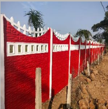
precast compound wall
