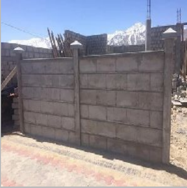
Rcc Compound Boundary Wall
