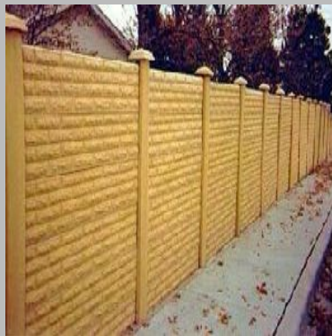
precast boundary wall
