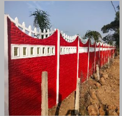
precast compound wall
