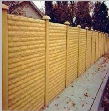
precast boundary wall
