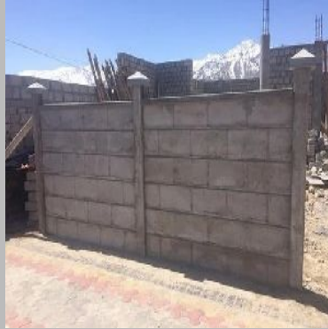
Rcc Compound Boundary Wall
