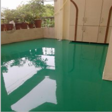
Roof & Terrace Waterproofing Service
