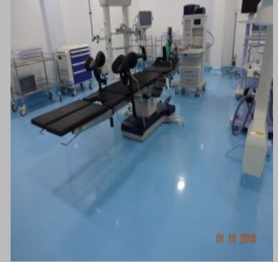
Industrial Epoxy Flooring
