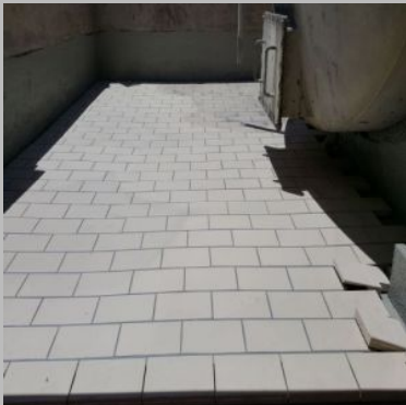
Acid Resistant Stone Brick Lining Service
