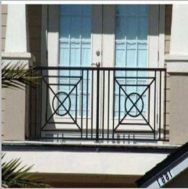
Mild Steel Balcony Railing
