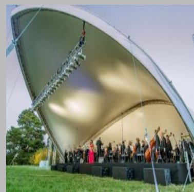
Membrane Structures Fabrication
