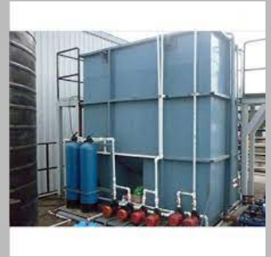
Packaged Sewage Treatment Plant
