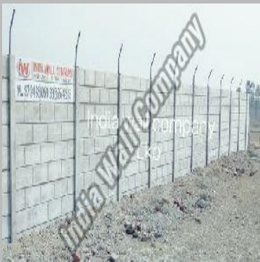
rcc compound wall
