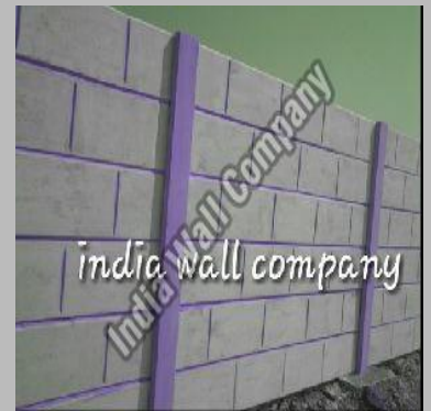
Precast Compound Wall
