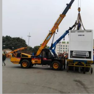
TRX Crane Rental Service
