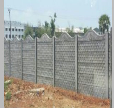
rcc compound wall
