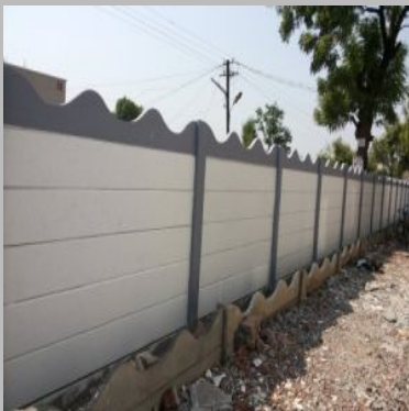
precast compound wall
