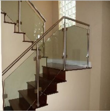
Stainless Steel Staircase Railing
