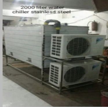
2000 Litre Water Chiller
