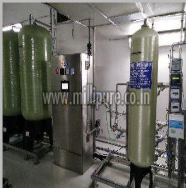
Demineralization Water Treatment Plant
