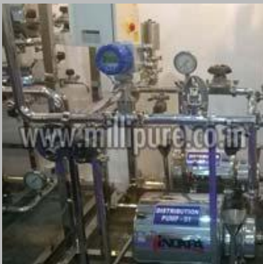
Purified Water Distribution System For PW / WFI
