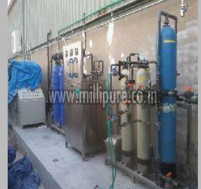
RO DM Water Treatment Plant
