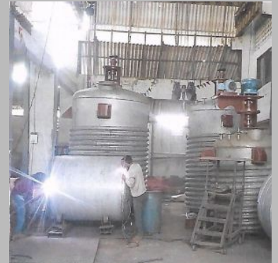
Chemical Reactor Vessel
