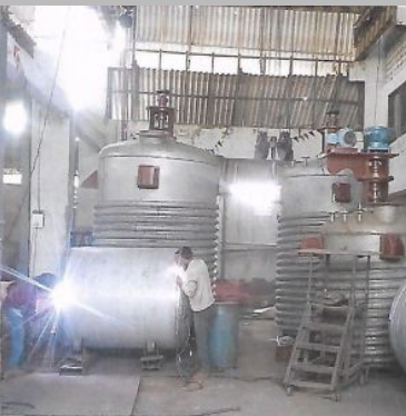
Chemical Reactor Vessel
