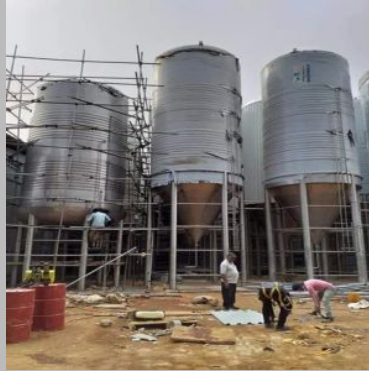
Dual Insulation Service
