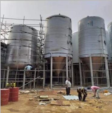
Dual Insulation Service
