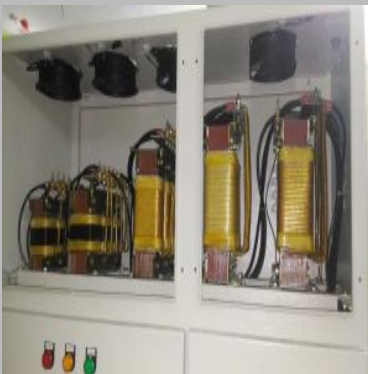
Detuned Harmonic Filter Panel
