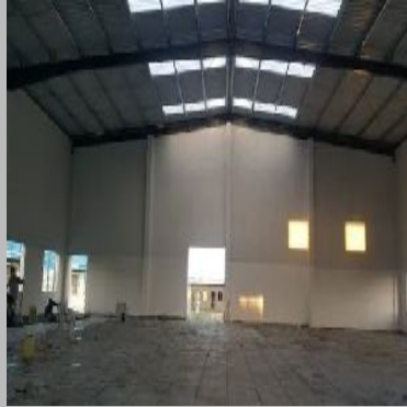
Prefabricated Roofing Shed
