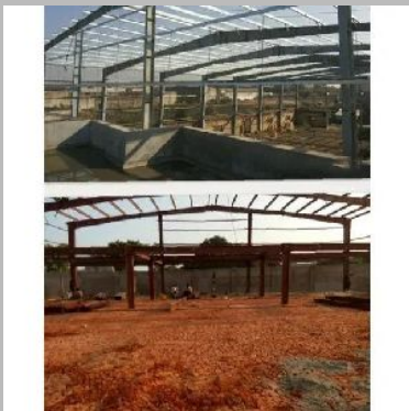
Badminton Court Roofing Shed
