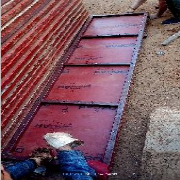
ms pipe shuttering frame
