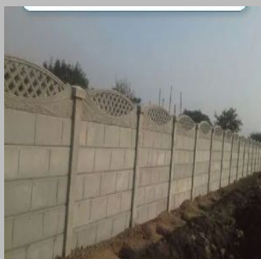
precast compound wall
