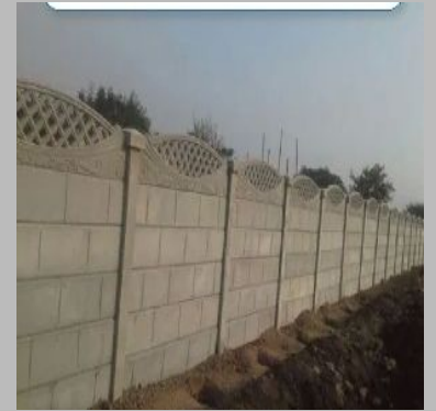
precast compound wall
