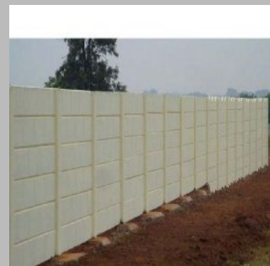
RCC Precast Compound Wall
