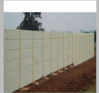
RCC Precast Compound Wall
