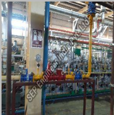
LPG High Pressure Gas Train
