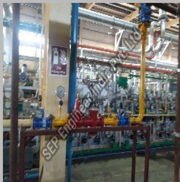
LPG High Pressure Gas Train
