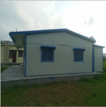
PUF Insulated Panel Building
