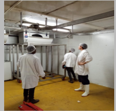
Cold Room Fabrication & Installation Service
