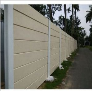
RCC Precast Compound Wall
