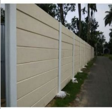
RCC Precast Compound Wall
