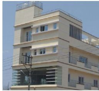
glass glazing work
