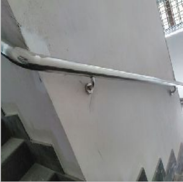
stainless steel stair railing
