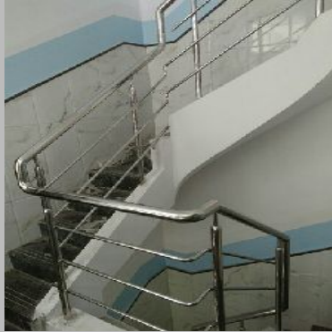
stainless steel railing works
