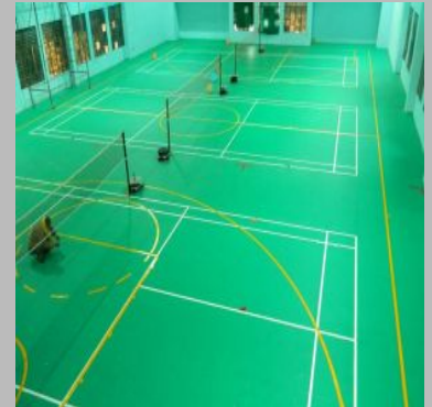
Basketball Court Flooring
