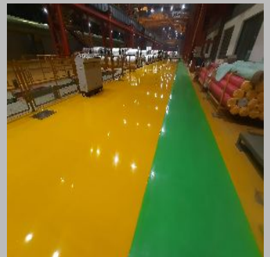
Epoxy Floor Coating
