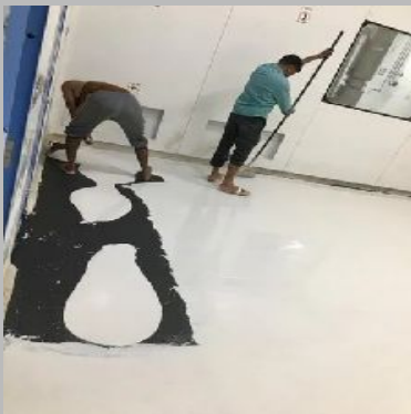
Staroxy ESD 1072 Epoxy Flooring Services
