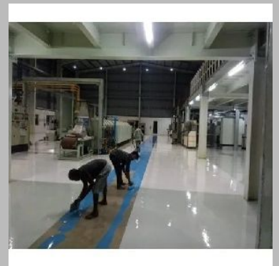
Commercial Epoxy Floor Coating Services
