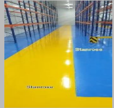
Topping PU Flooring Services
