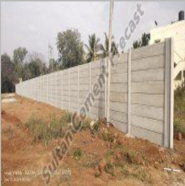
Precast Concrete Compound Wall
