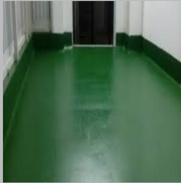
pu flooring services
