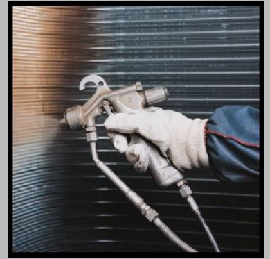
Anti Corrosive Coating Services
