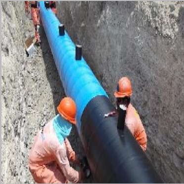
Pipeline Coating Services
