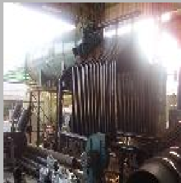
Steam Boiler - Membrane Type
