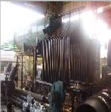
Steam Boiler - Membrane Type
