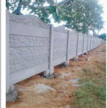
RCC Precast Compound Wall
