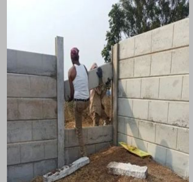
RCC Precast Boundary Wall Installation Service
