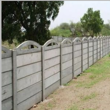
Concrete Readymade Boundary Wall
