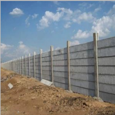
Concrete Readymade Compound Wall
