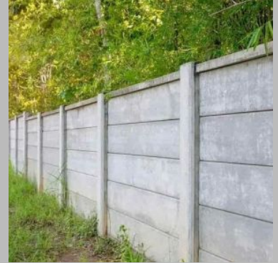
RCC Precast Boundary Wall
