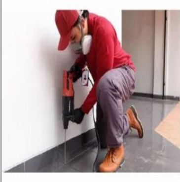
Post Construction Anti Termite Treatment Service
