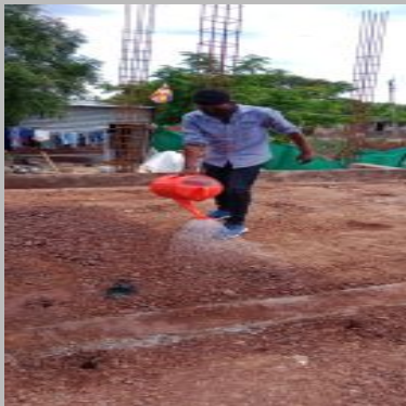
pre contraction anti termite treatment
