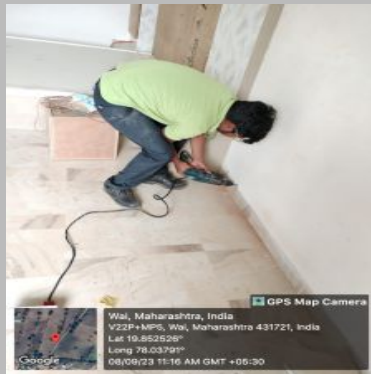
Post Contraction Anti Termite Treatment
