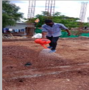
pre construction anti termite treatment
