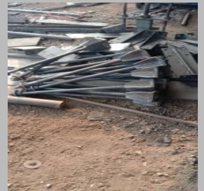
Plate type foundation bolt with stiffner
