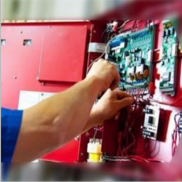
Fire Alarm System Repairing Services
