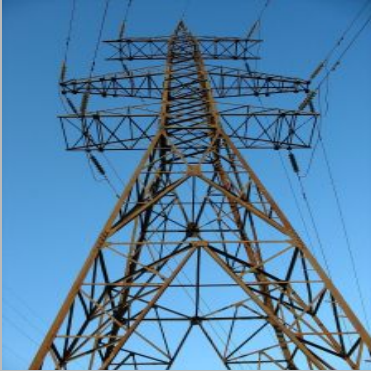
Transmission Line Construction Service
