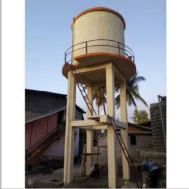
Water Tank Construction Services
