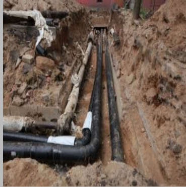
Sewer Pipeline Construction Service
