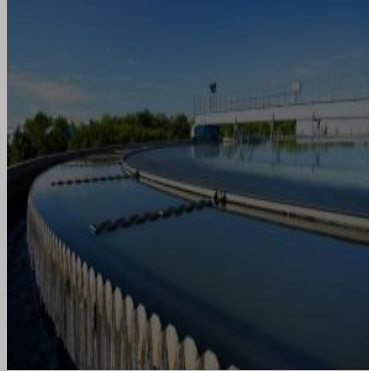
Water Reservoirs Construction Services
