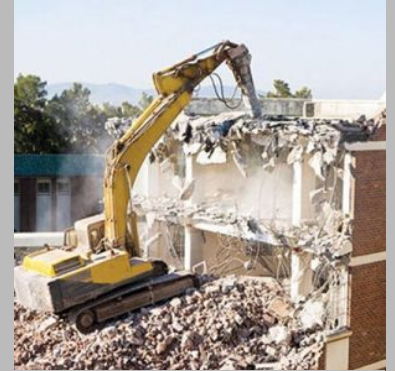
Building Demolition Services
