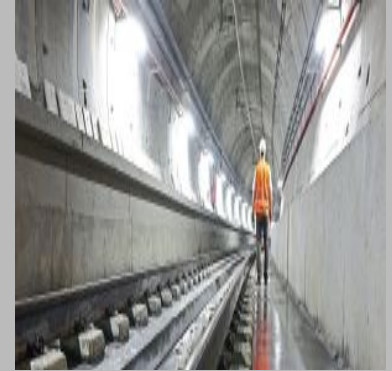
Tunnel Construction Service
