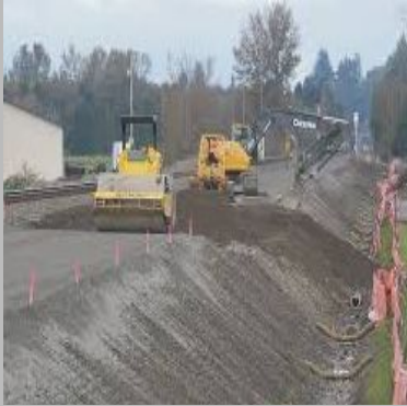
Railway Siding Works
