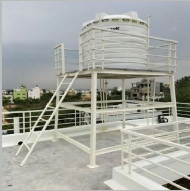
Iron Water Tank Stand
