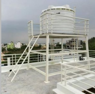
Iron Water Tank Stand
